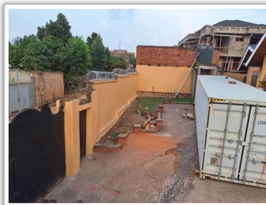
Outer Wall - Fence Repaired
